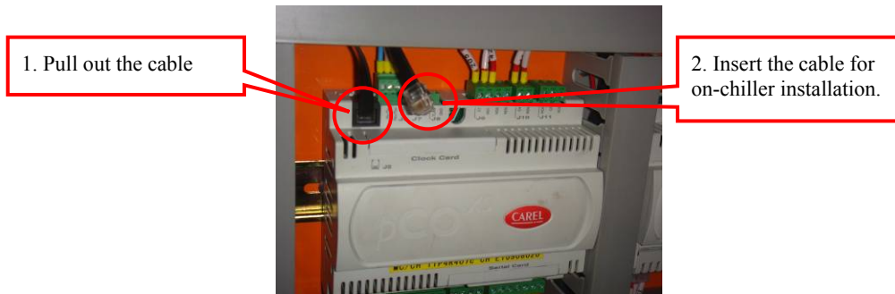
Fig.- 18 Remote controller cable connecting with controller
